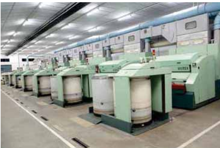
A view of Rieter C60 Carding Machines installed at our unit Rajapalayam Spintext.
